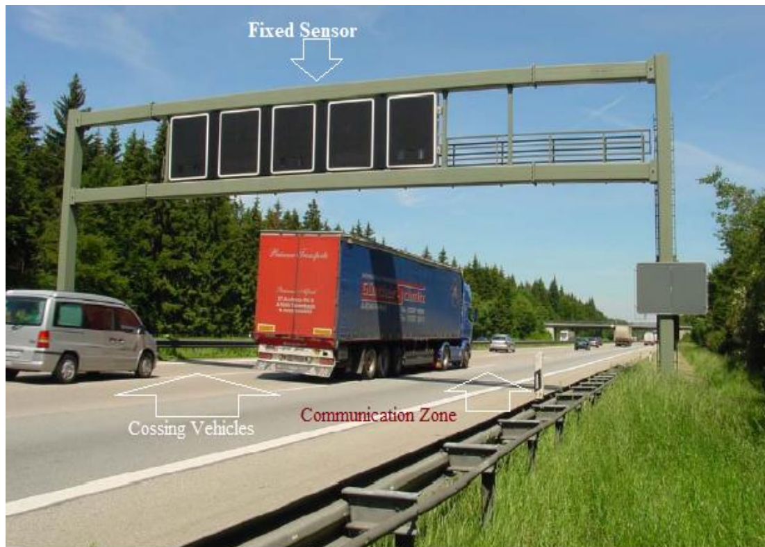
Figure 2.6: Traffic Source Data; Point Sensor. (Dutch National data, 2018)
